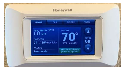
Honeywell Prestige Color Thermostat (8 in Main House; 3 in Guest House)
